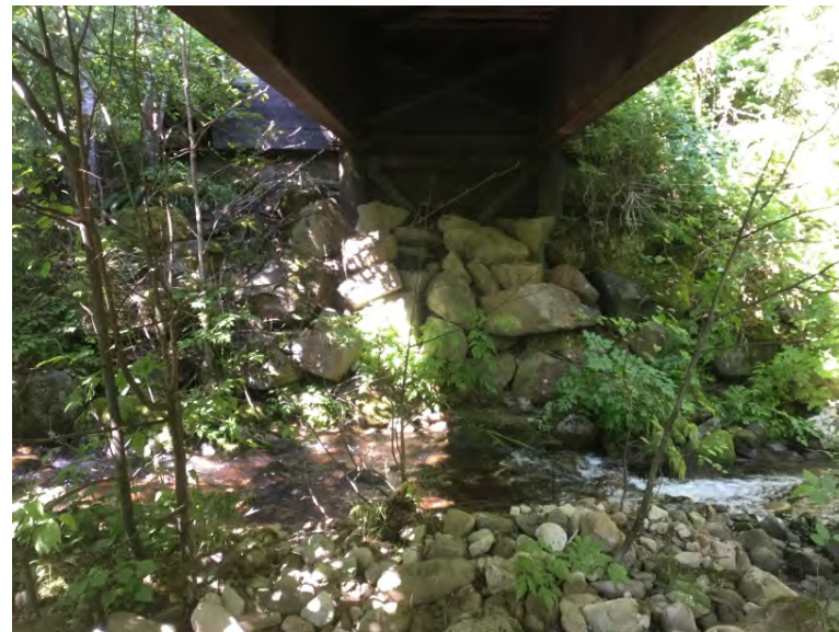
Left Bank Abutment when facing downstream
