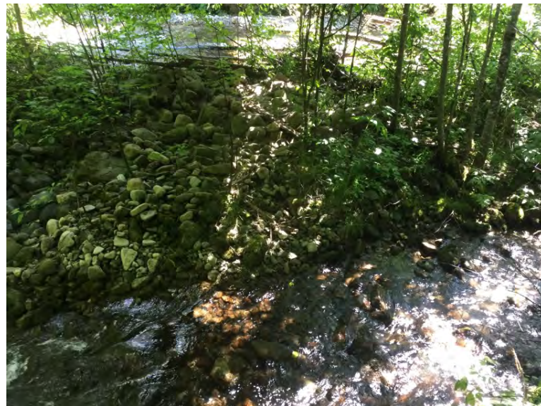
2 stream channels under bridge
