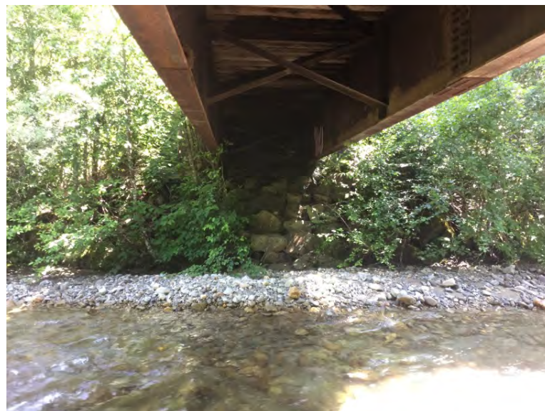
Right Bank Abutment when facing downstream
